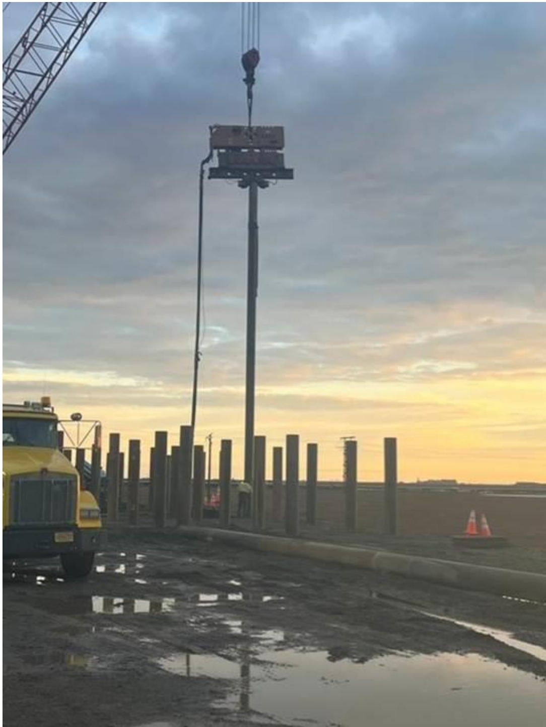
Workers and project partners celebrate the installation of the final foundation pile at the Alyeschem chemical and fuels manufacturing facility in Prudhoe Bay, marking another major construction milestone as development of Alaska's first Arctic petrochemical facility continues. Photo taken September 12, 2026, by Alyeschem.
