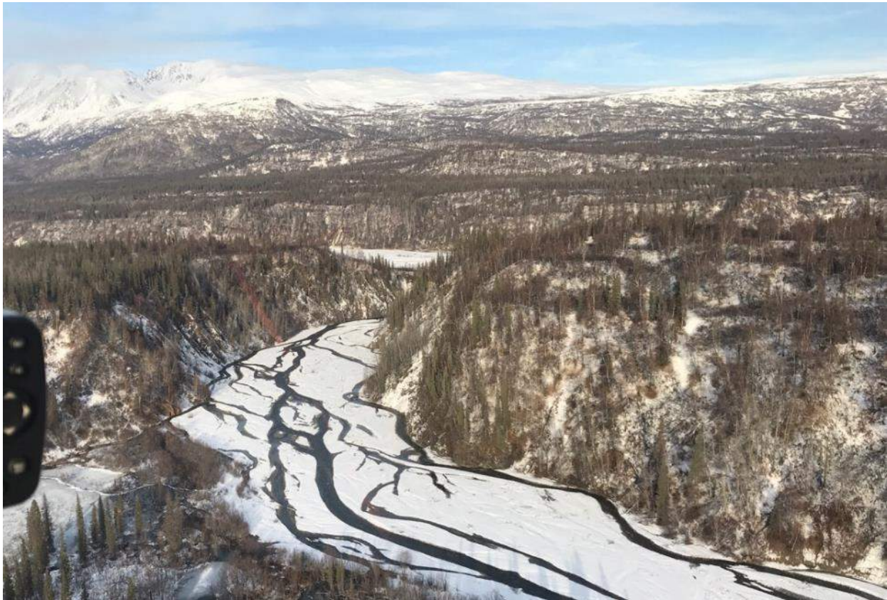
Figure 10: Old Man Creek (looking downstream). Note the steep canyon where the proposed bridge crossing would be located. This bridge would be approximately 1,000 feet long.
