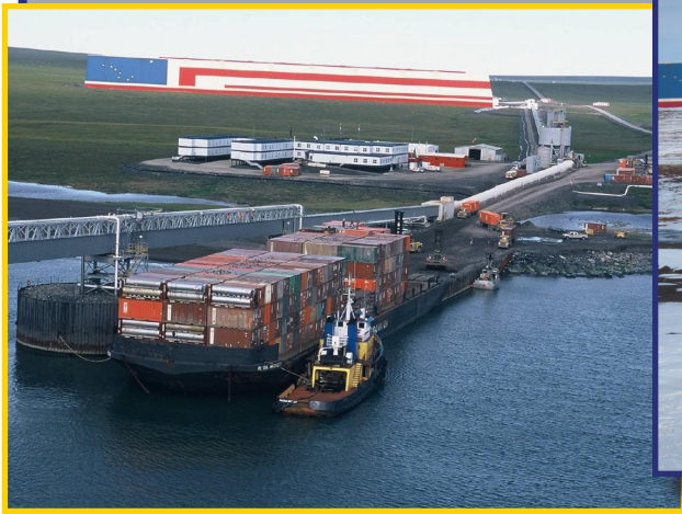
Photo of the shiploader and conveyor with incoming supplies and container barge
