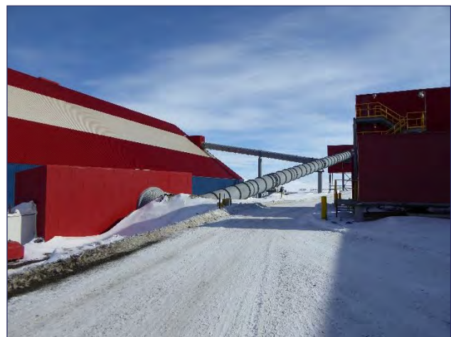
CSB#2 and concentrate conveyor to shiploader
