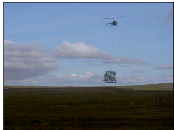
Snowfence being installed along DMTS road, 2007
