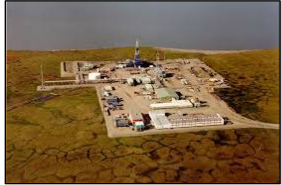
Badami production facilities (ADN 2014)
