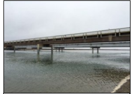
Sagavanirktok River West Channel Bridge (WERC 2025)
