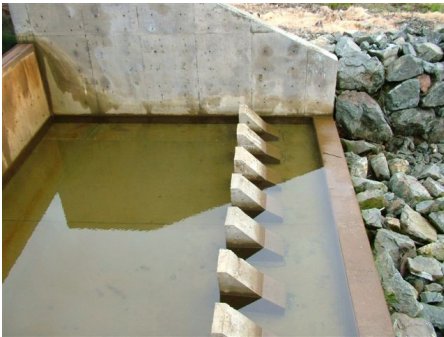
Diversion structure for South Fork hydro project
