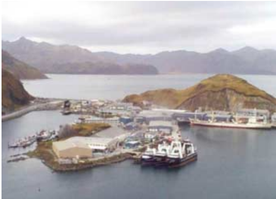
Figure 01 - UniSea Seafood Processing Facility at Unalaska/Dutch Harbor, Alaska
